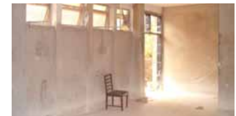
One of the freshly plastered new theatres
